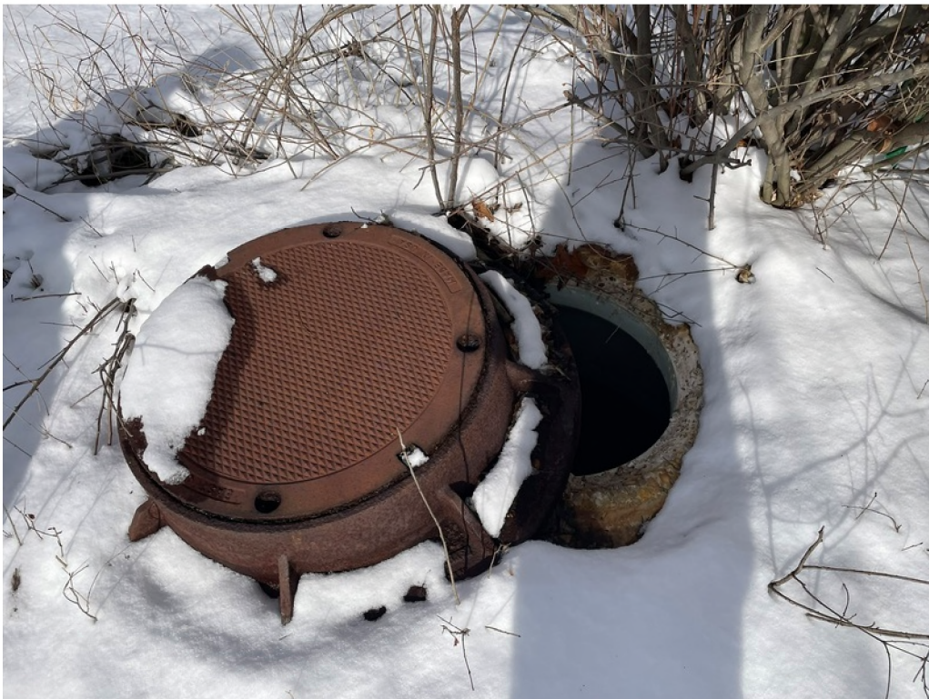
Sewer manhole cover in northwestern portion of subject property
