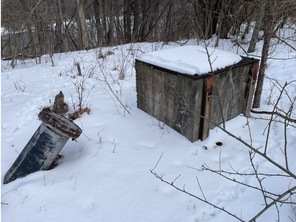
Capped pipeline in northern portion of subject property
