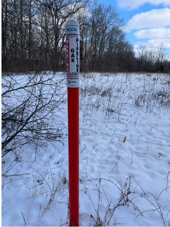
Gas pipeline marker in the northern portion of subject property
